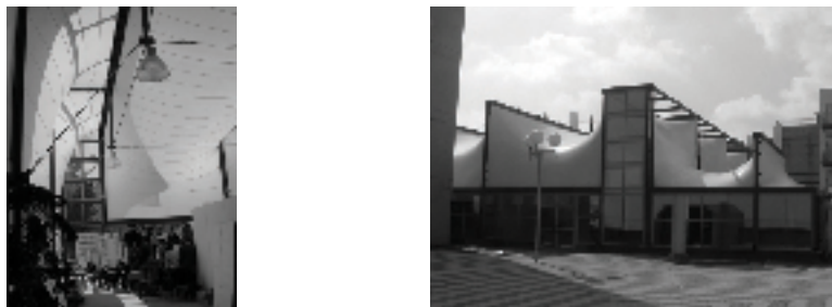
Fig. 4 – Amado roof membrane structure
