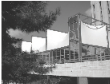
Figure 5: The Amado membrane roof structure – the overall orthogonal assembly composition of rigid-edge membrane units.
